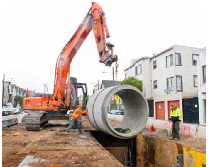
New conveyance pipe on Cesar Chavez St in the Mission District
