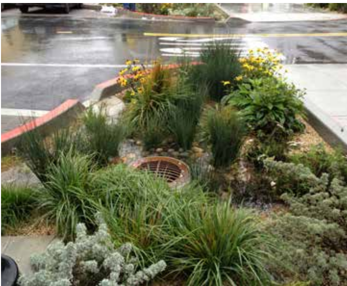
Rain garden on Newcomb Avenue in San Francisco's Bayview Neighborhood
