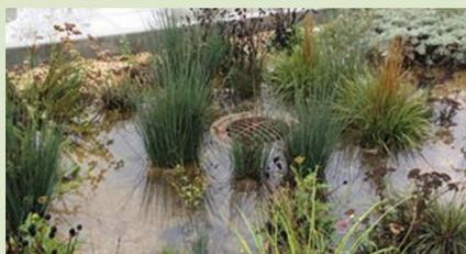
**Rain Gardens:** Capture stormwater runoff from streets, roofs, and parking lots. Plants and soil absorb that water, reducing the amount of runoff overwhelming the sewer system.
