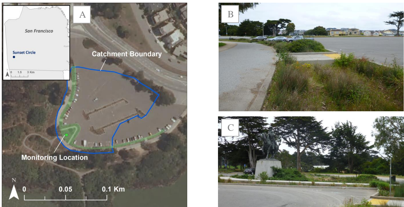
Figure 1. A) Aerial view showing location of Sunset Circle vegetated swales and infiltration basin system, with GI features shaded in semi-transparent green along the edge of the u-shape, B) View of vegetated swales lining parking lot, and C) View of large infiltration basin and statue.
