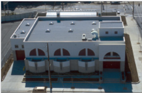
Figure I-13. Bruce Flynn Pump Station
