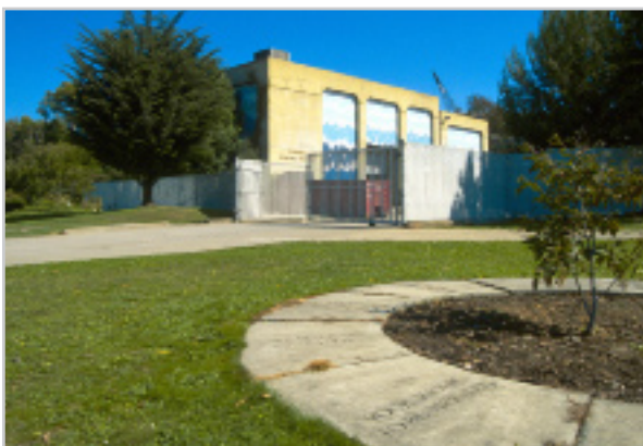
Figure I-3. Channel Pump Station
