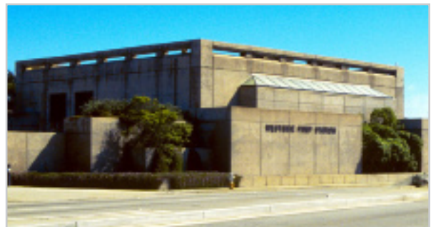
Figure I-10. Westside Pump Station
