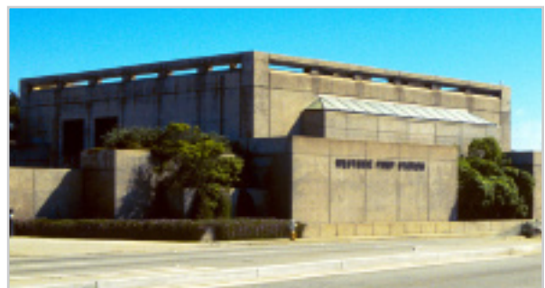
Figure I-10. Westside Pump Station
