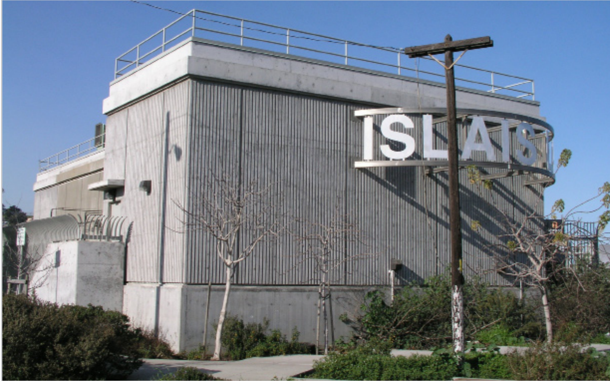
Figure I-17. Booster Effluent Pump Station
