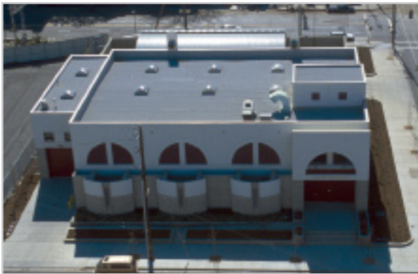
Figure I-13. Bruce Flynn Pump Station
