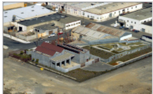
Figure I-7. Griffith Pump Station
