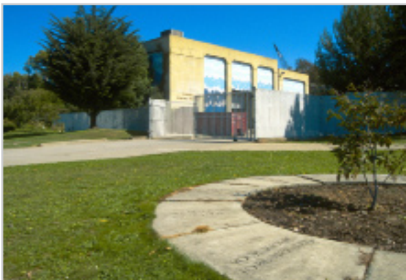
Figure I-3. Channel Pump Station
