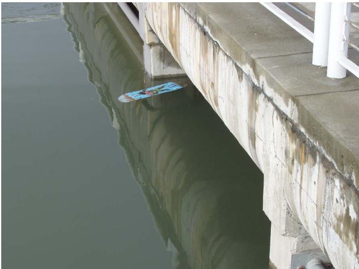
**FIGURE 5A. BACKFLOW OF BAY WATER INTO A COMBINED SEWER DISCHARGE STRUCTURE**
