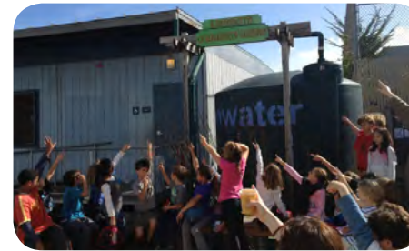
Lafayette Elementary's Rainwater Harvesting System
