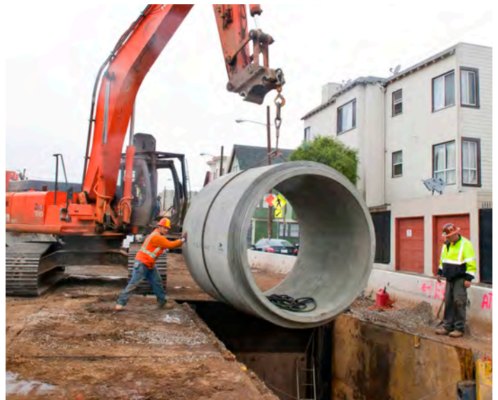
Conveyance pipe construction.
