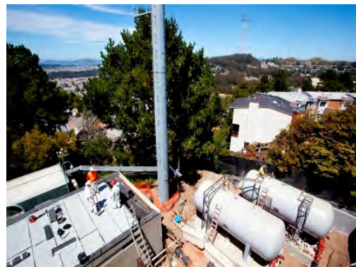
Construction of Forest Hill Pump Station and Hydro-pneumatic Tanks
