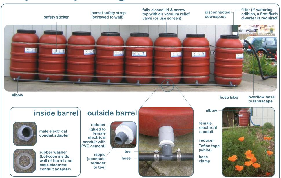
A daisy chain system is an alternative to a cistern, and an easy way to expand on a single rain barrel system in order to capture more water. The photos above show a rainwater harvesting demonstration project at the San Francisco Public Utilities Commission Southeast Treatment Plant. For more information, email greenstormwater@sfwater.org.
