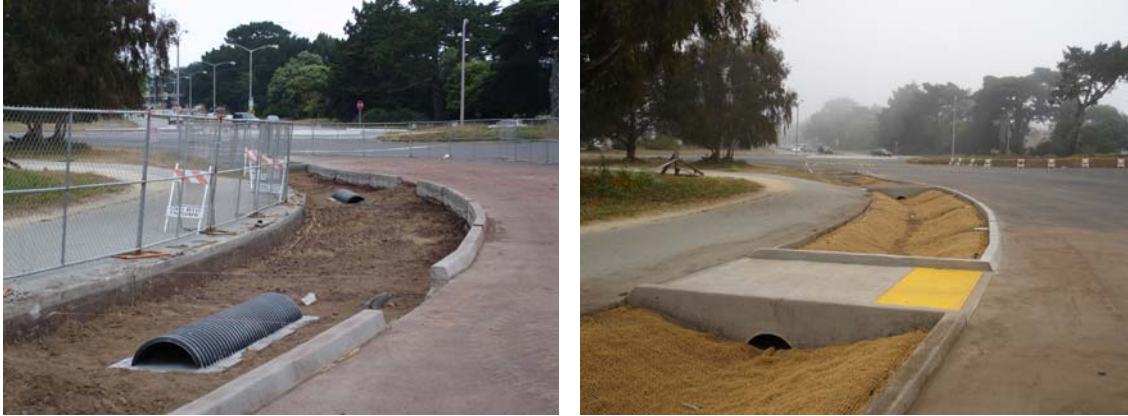
Photos from Construction
