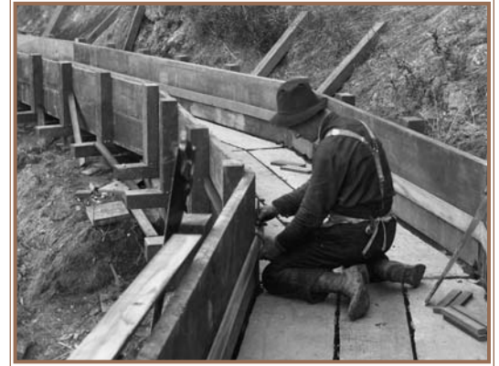
Construction of Stone Dam Flume 1871
