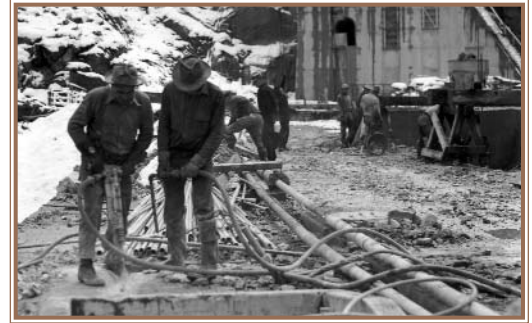
Roughening the crest of O'Shaughnessy Dam 1937
