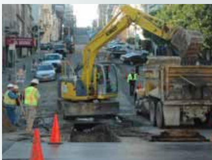
Before: Webster and Union streets during water and sewer main construction.
