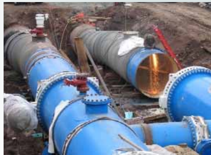
Bay Division Pipeline #4 construction.
