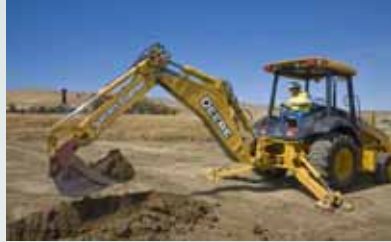
Digging the footprint for the new Tesla Water Treatment Plant.
